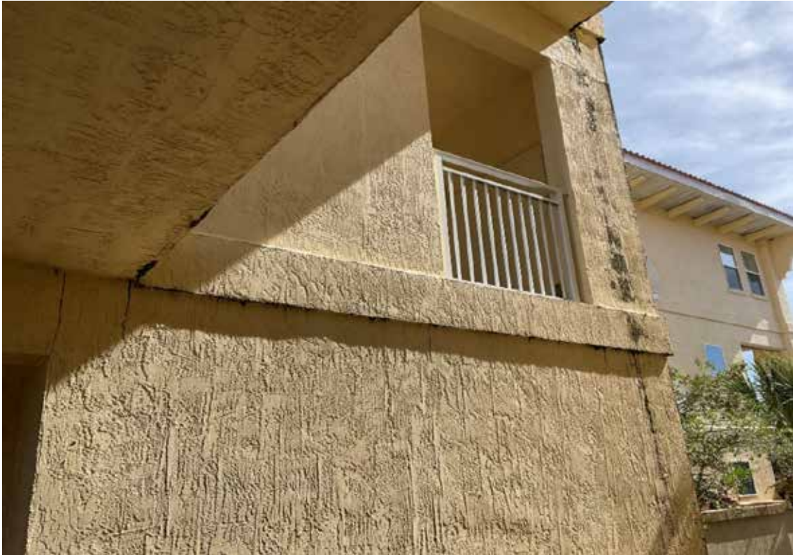
Bldg 300 - Paint Condition
