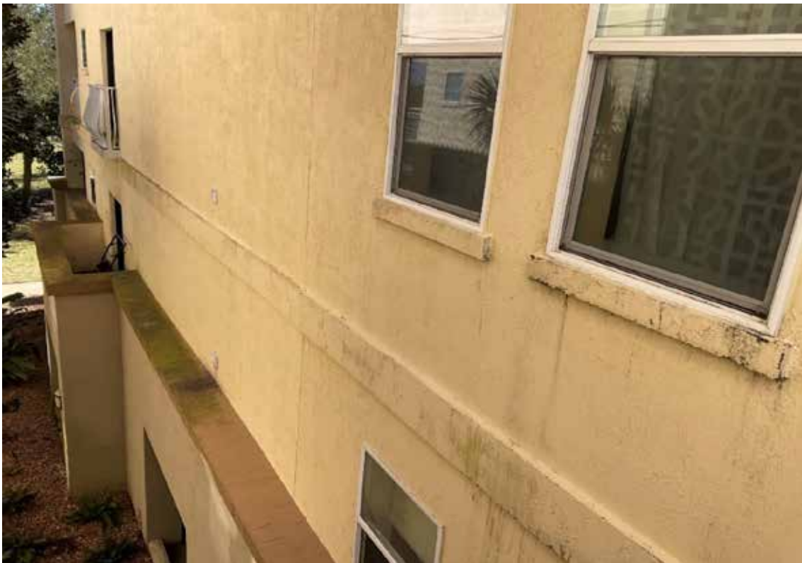
Bldg 100 - Paint Condition
