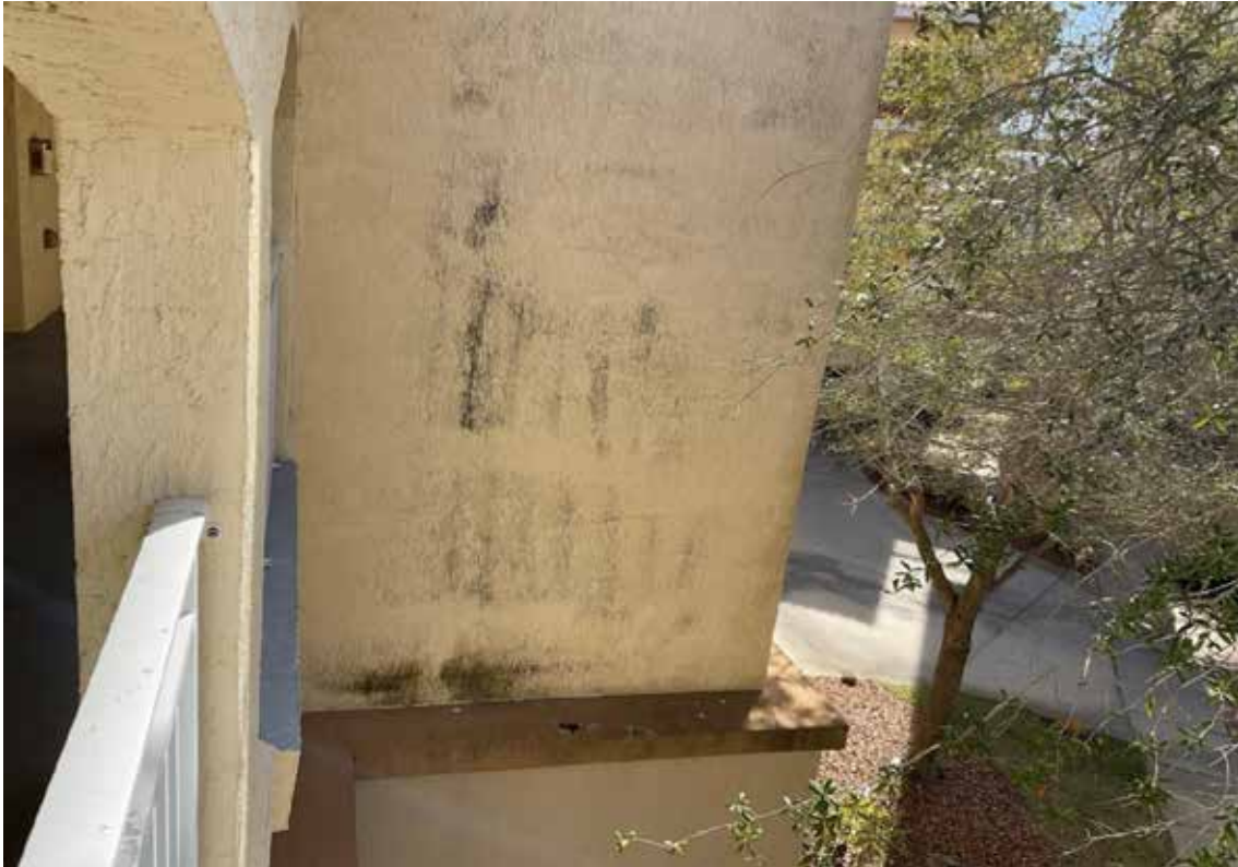
Bldg 200 - Paint Condition
