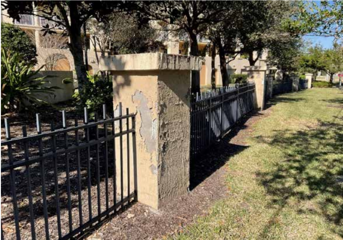
Fence & Columns - Property Line
