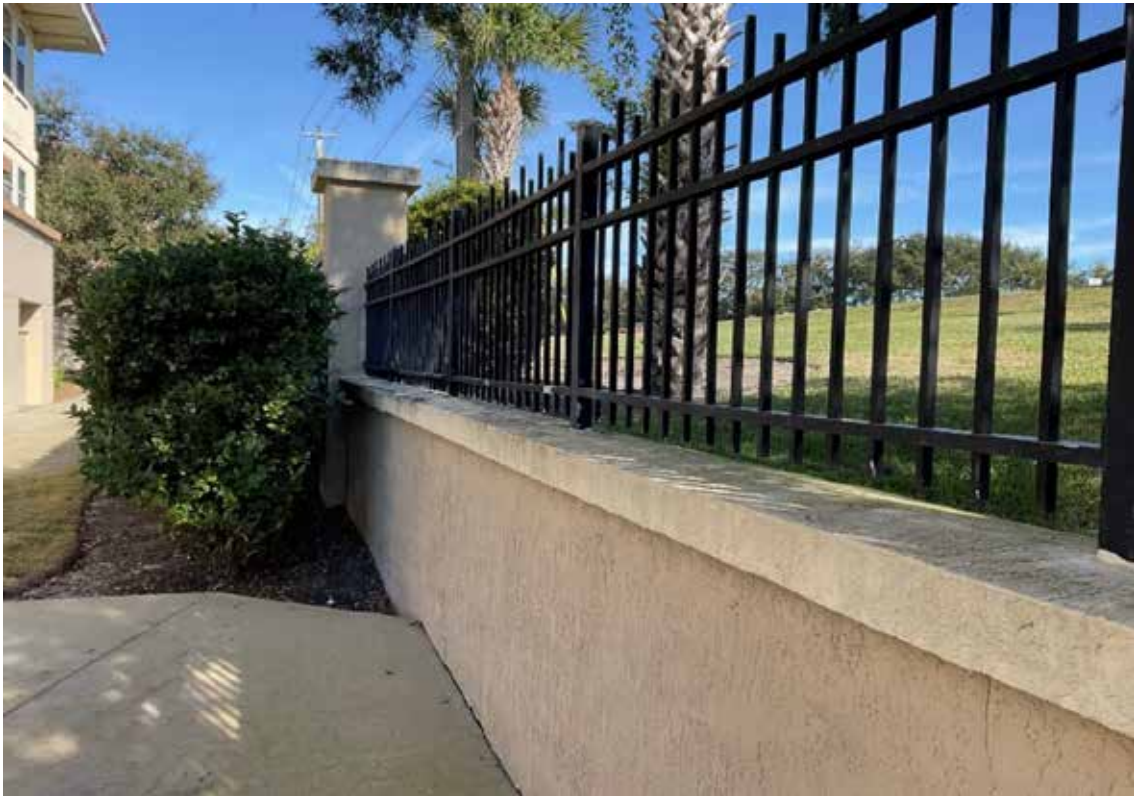
Retaining Wall & Fence
