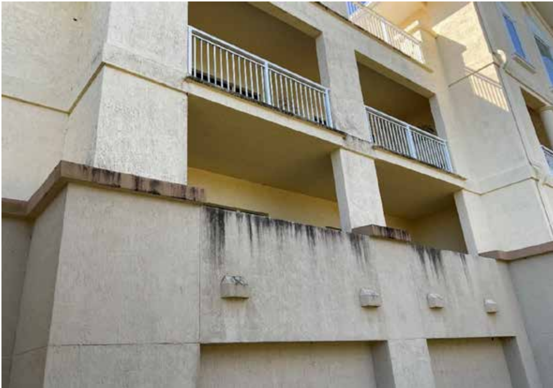
Bldg 200 - Paint Condition
