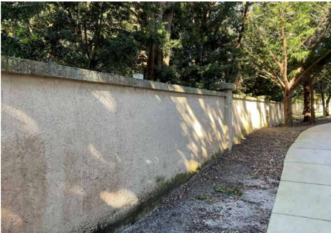
Site Wall - Property Line
