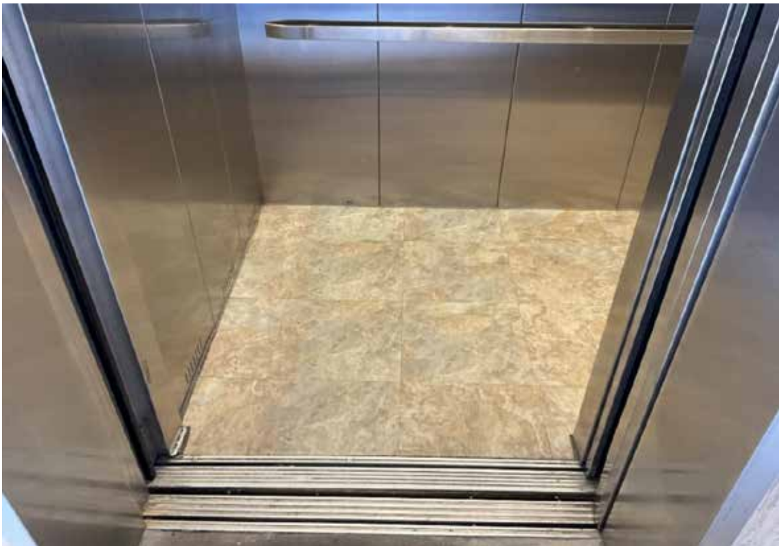
Bldg 100 - Elevator Cab
