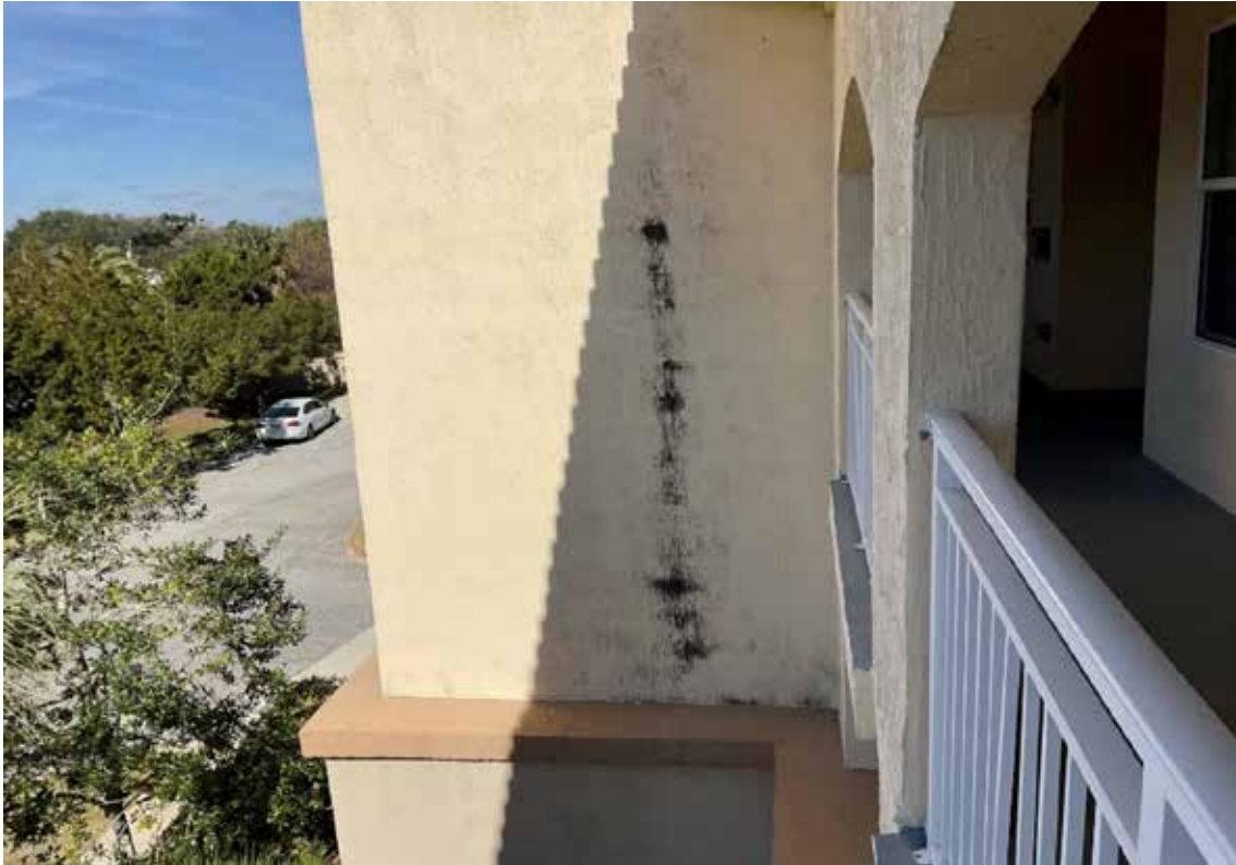
Bldg 100 - Paint Condition
