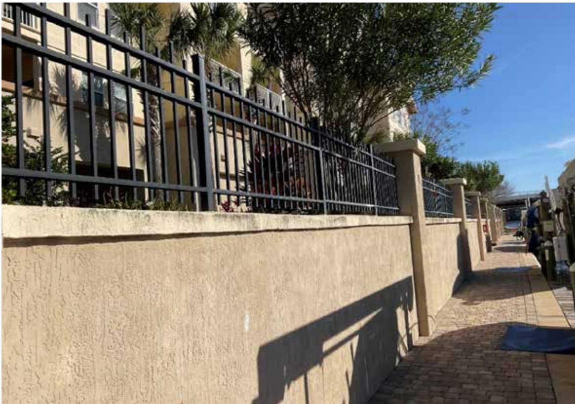
Retaining Wall & Fence
