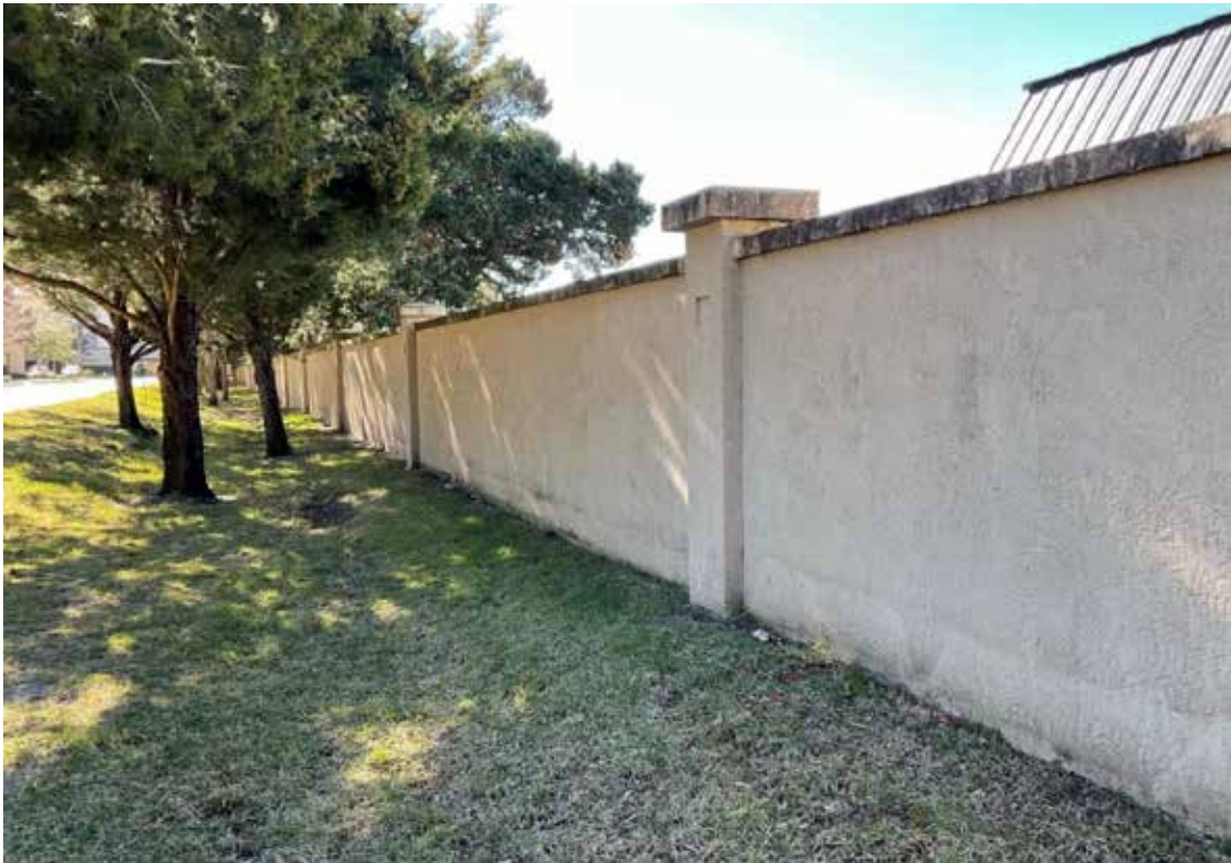
Site Wall - Property Line
