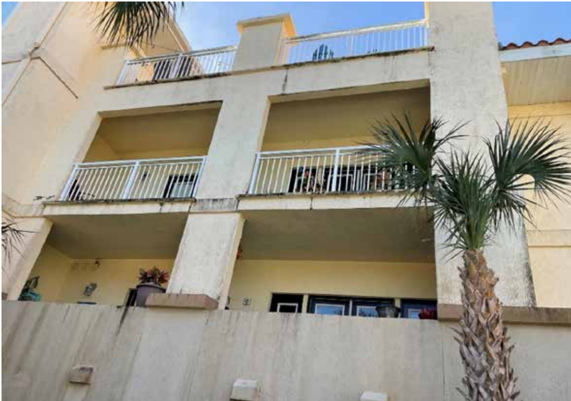
Bldg 200 - Paint Condition
