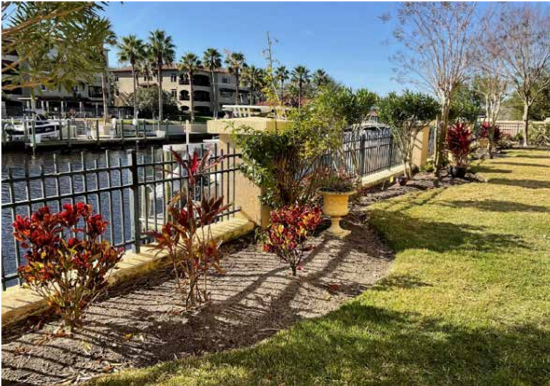
Retaining Wall & Fence
